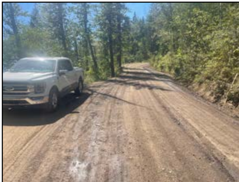
4 – Freshly graded and treated section of Hartley Lake Road for dust control near resident homes, in partnership with RDEK, TC Energy & SMJV who donated the man-power and machinery in 2022 for the work needed.
