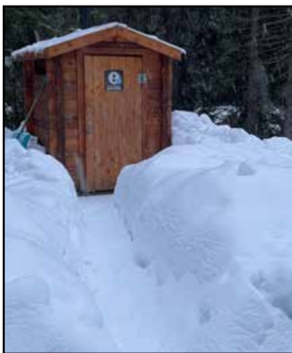
Pathway cleared for when you've got to go! The AmbassadorWILD™ program helps maintain the toilets in Mt Fernie Provincial Park during winter.
