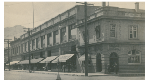
3 THE HOME BANK 491 2nd Avenue
